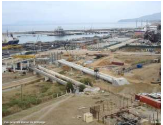
Ø 2000 mm: Skikda (Algeria) Free span of 26m
