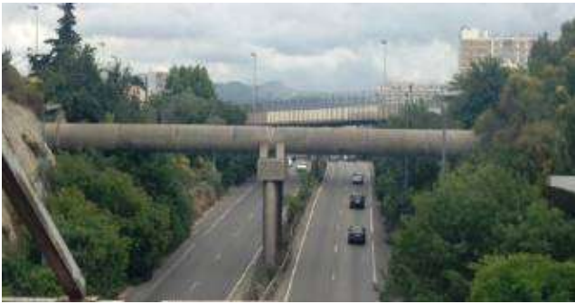
Ø 1800mm : Marseille (France) Free span of 20m
