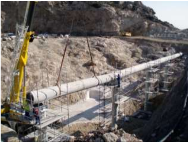
Ø 800: Marseille (France) Free span of 12,3m
