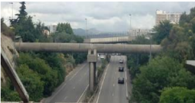
Ø 1800mm : Marseilles (France) Free span of 20m
