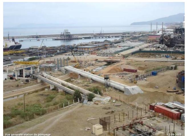
Ø 2000 mm: Skikda (Algeria) free span of 26m test pressure: 6b
